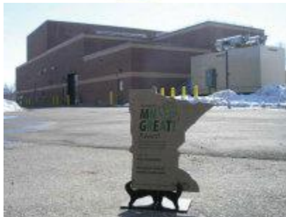
The Mankato Water Reclamation Facility
