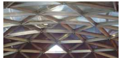
Underside view of skylights
