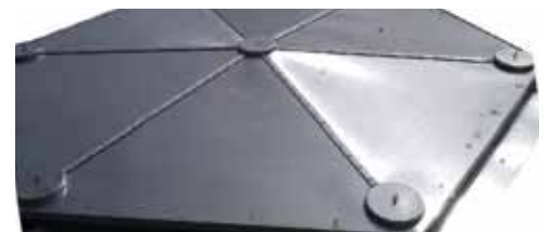
Large hatch for equipment removal
